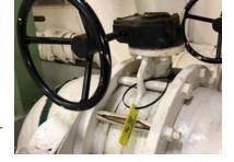
UHF tag version with fixed readers or UHF enabled mobile scanning devices for inventory/shipping/receiving workflow automation.
